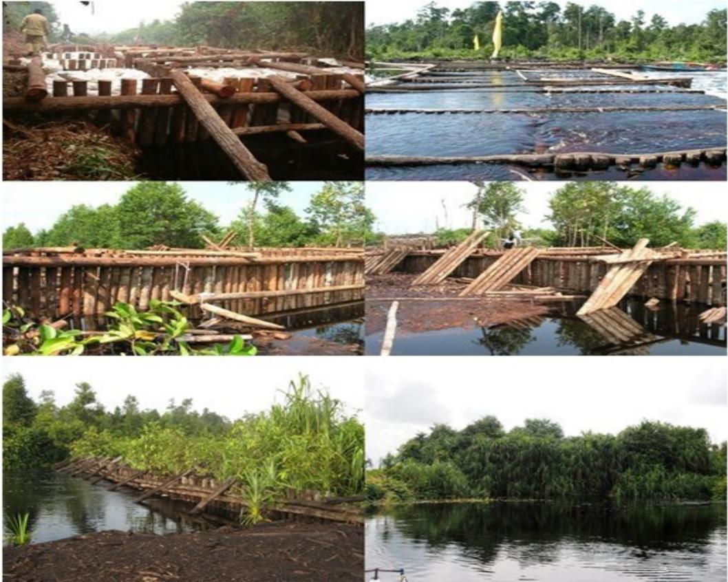
**GAMBAR 16** | Contoh gambar Sekat Kayu Multi-Lapis tanpa Peluap (Non-spillway)
