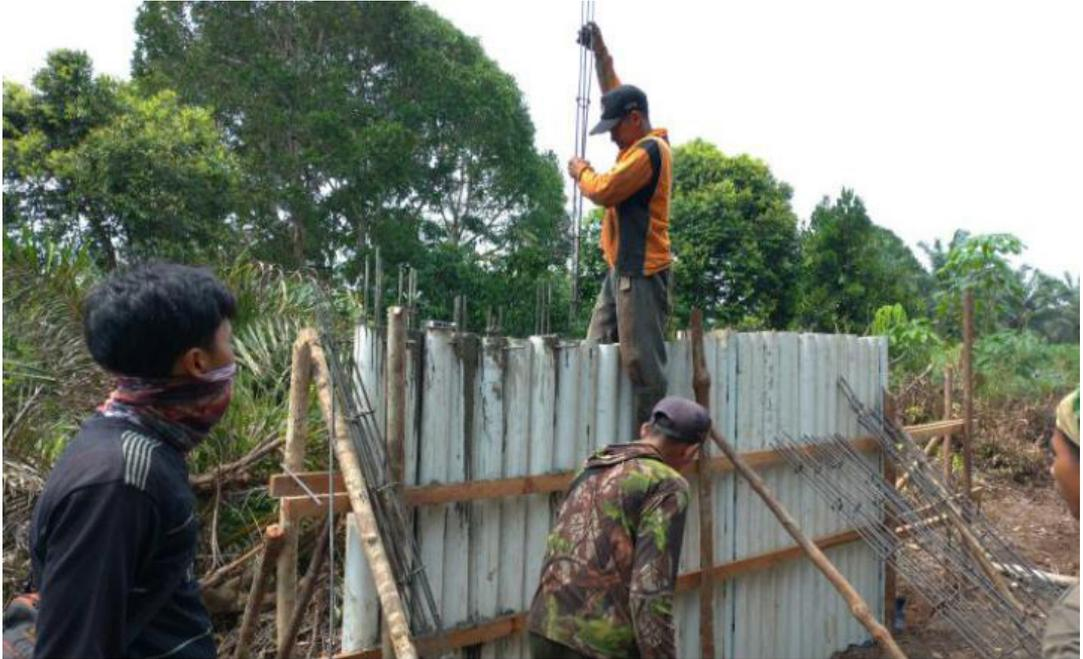
**GAMBAR 60** | Pembesian Pipa PVC Beton
