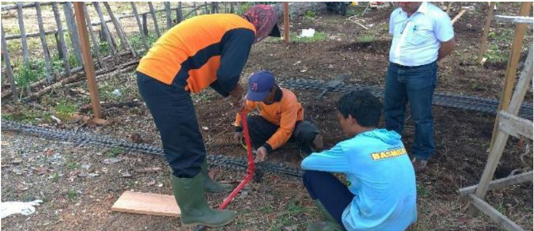
**GAMBAR 84** | Pembesian *Hollow block*
