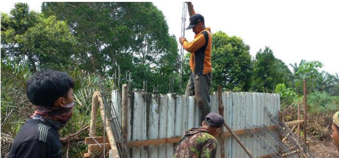
**GAMBAR 85** | Pembesian pipa PVC beton
